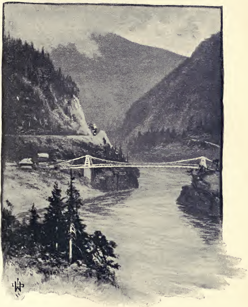
CARIBOU ROAD BRIDGE, FRASER.
